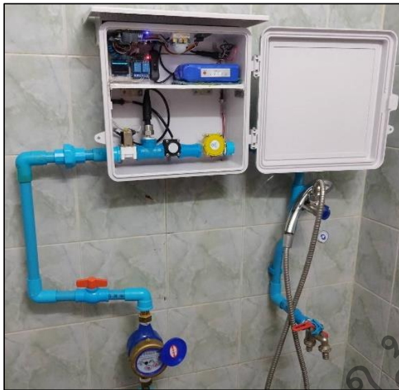
Fig. 7 Examples of installation and testing in real-world settings.
